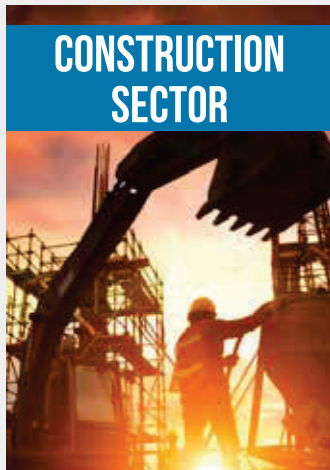
Temporary datacenter for big construction sites ( ports , airport )
